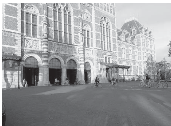
Figure 1 Rijksmuseum and its underpass (northern façade)
